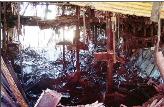
Figure 1: Internal collapse area in WTC 5 [1]
